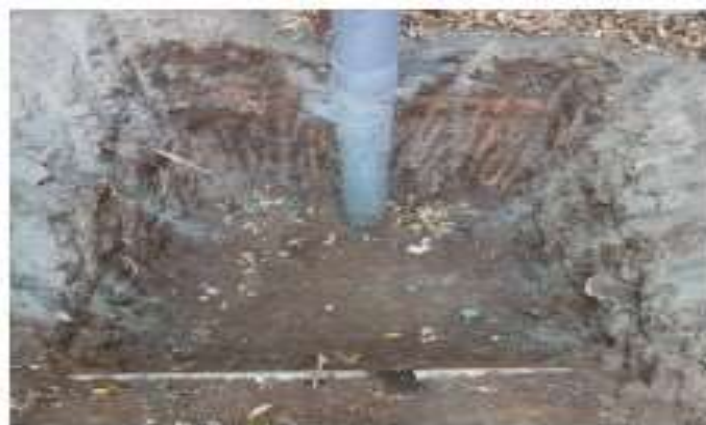
Figure2a: Excavation at the site
