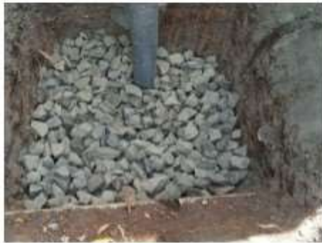
Figure2b: Layers of 40mm Boulders
