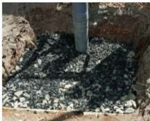
Figure2d: Layer of Charcoal
