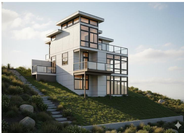
Figure 1: An Indicative RC Structure positioned on inclined ground
