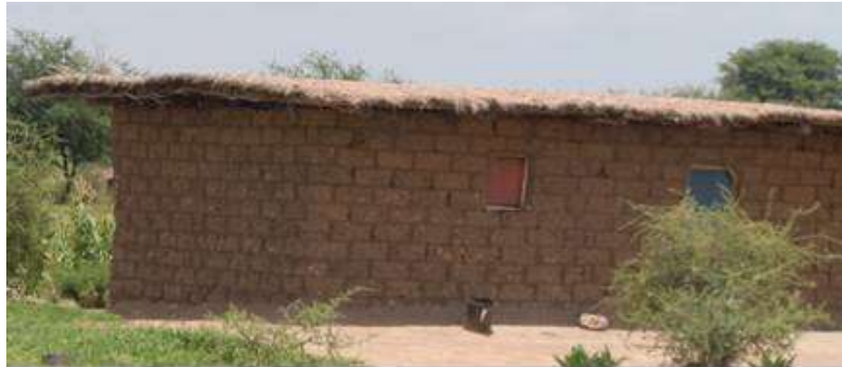
Figure 2: Soil brick house thatched with grass.
