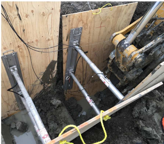
(c) Hydraulic shoring protection system retain the sensitive clay soil pressure
